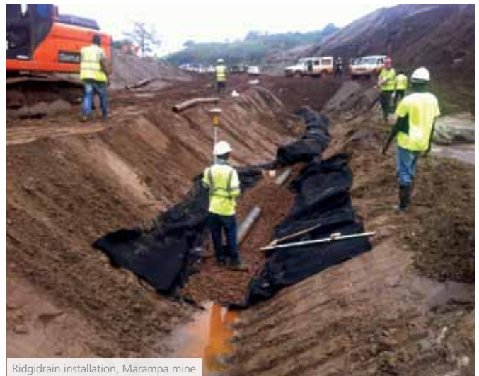
Ridgidrain installation, Marampa mine
