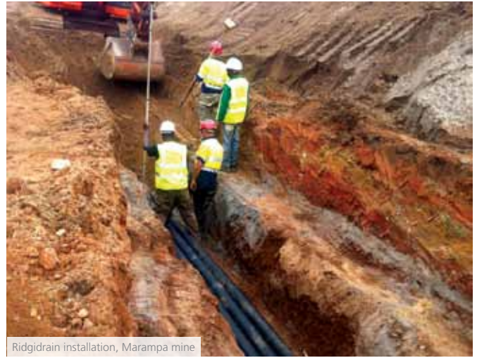
Ridgidrain installation, Marampa mine
