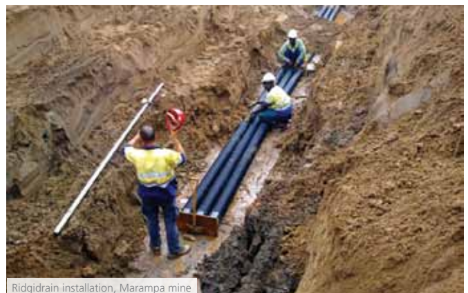
Ridgidrain installation, Marampa mine
