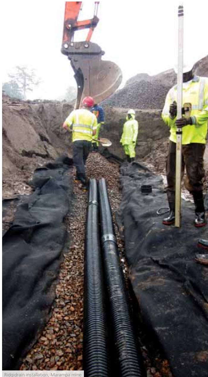
Ridgidrain installation, Marampa mine
